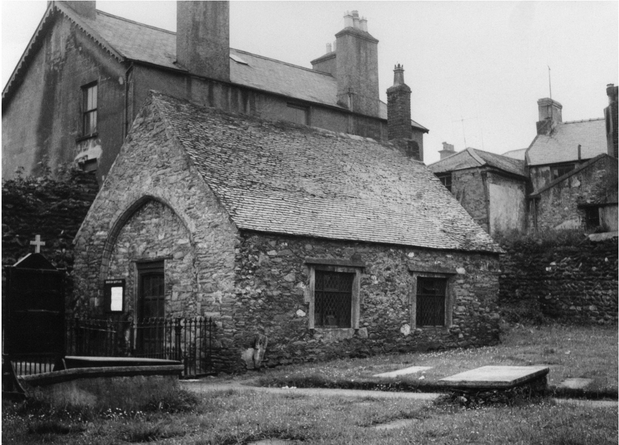
Photo of Eglwys Y Bedd from 1954, showing the graveyard and infilled chancel archway; image from Coflein.
